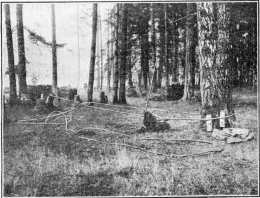
FIG. 8.—Pulling a second-growth fir stump by means of a hand stump puller.
